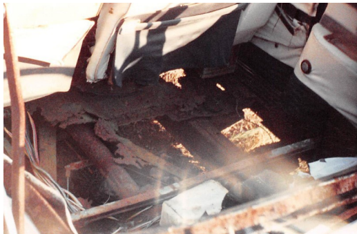
Floor panels completely rusted through.
